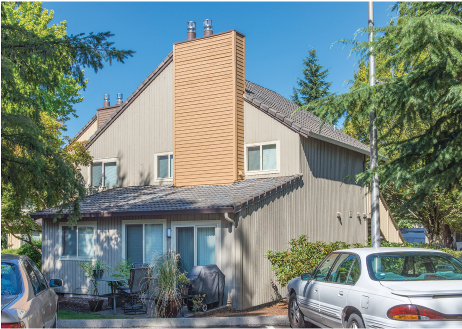
Nobl Park in Vancouver, WA, features 144 high-efficiency natural gas fireplaces, which provide affordable, clean heat for about 40 cents an hour.
