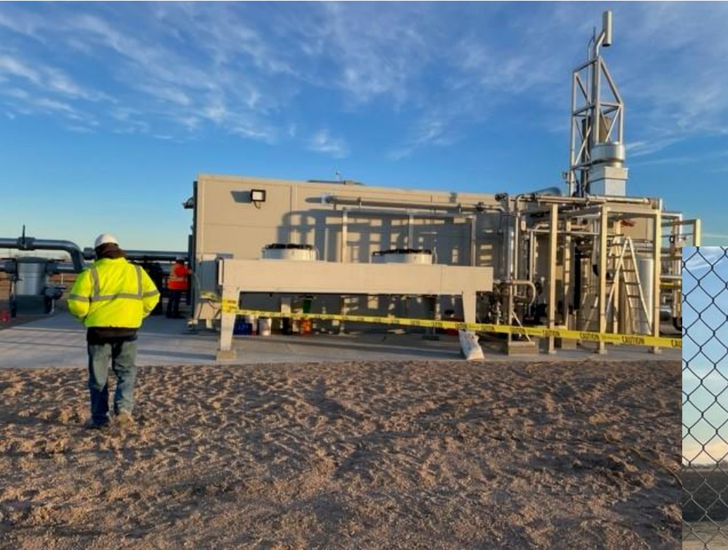
Gas cleaning skid
