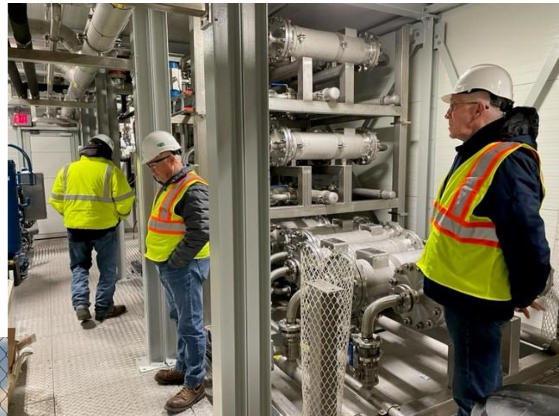
Inside of skid (membranes visible)
