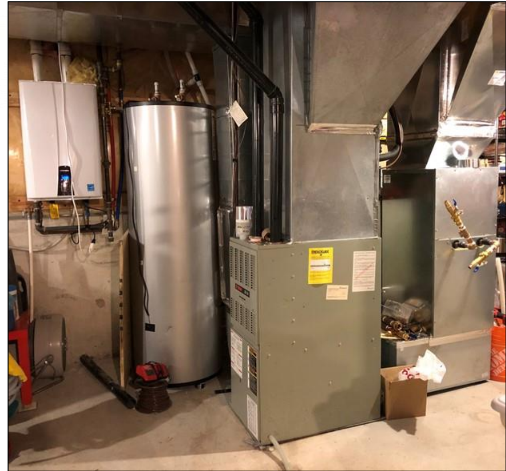
GHP water heater
